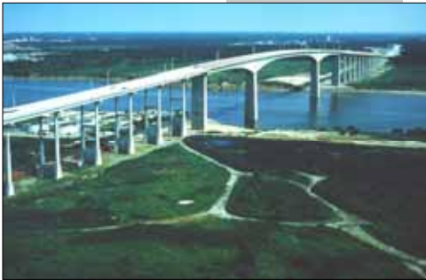
Houston Ship Channel Bridge
